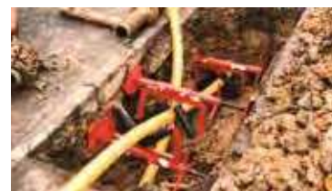
PRT1 - Pipe Roller for trenches
